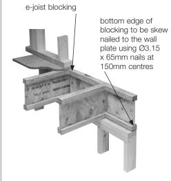
note: use for sub-floor and upper floor blocking on either single or multi-storey construction
