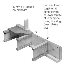
note: double rimboards for the lower storey of two storey construction
