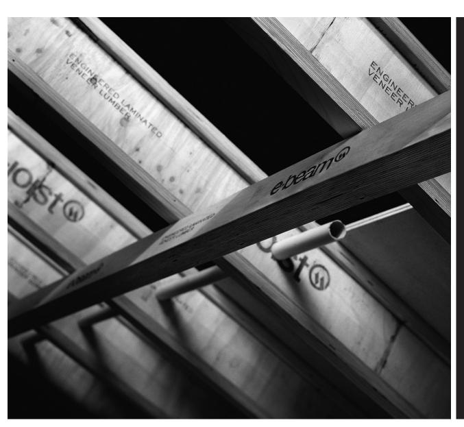
engineered floor joists
